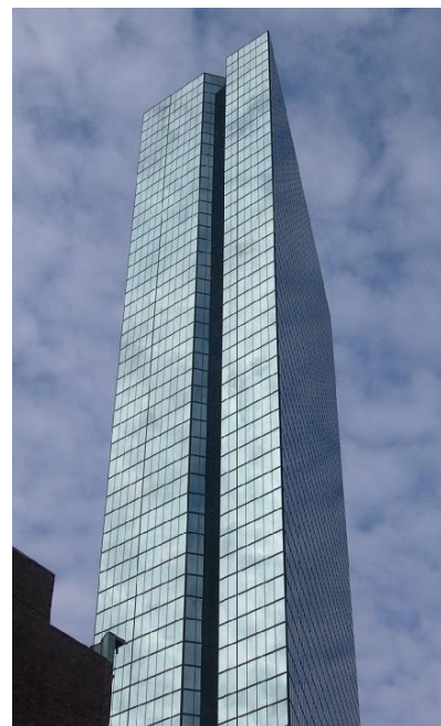
c / The John Hancock Tower in Boston vibrates naturally at a frequency of 0.14 Hz. Surprisingly, this frequency is the same regardless of the amplitude of the vibrations
